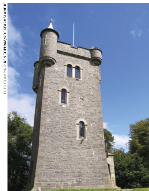
Helen's Tower, county Down, Irish Landmark Trust
