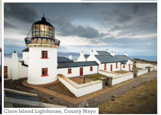
Clare Island Lighthouse, County Mayo
