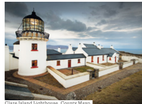
Clare Island Lighthouse, County Mayo
