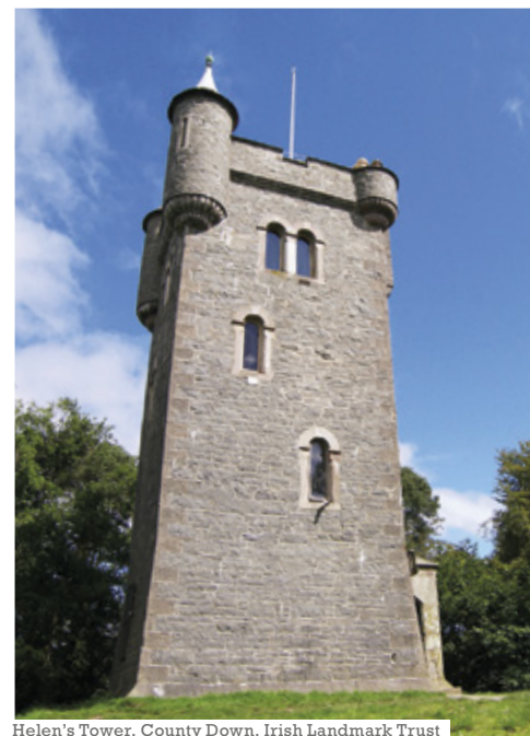
Helen's Tower, County Down, Irish Landmark Trust
