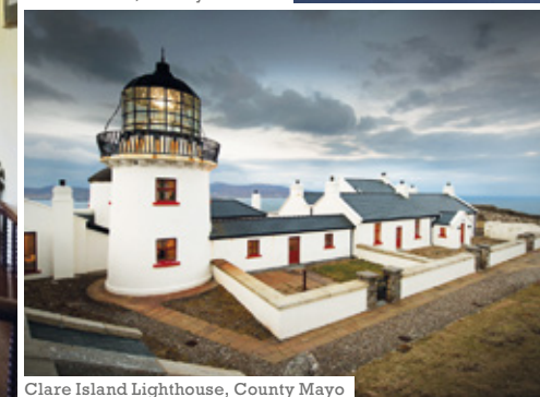
Clare Island Lighthouse, County Mayo
