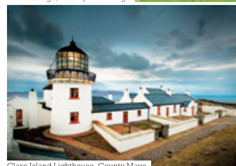
Clare Island Lighthouse, County Mayo
