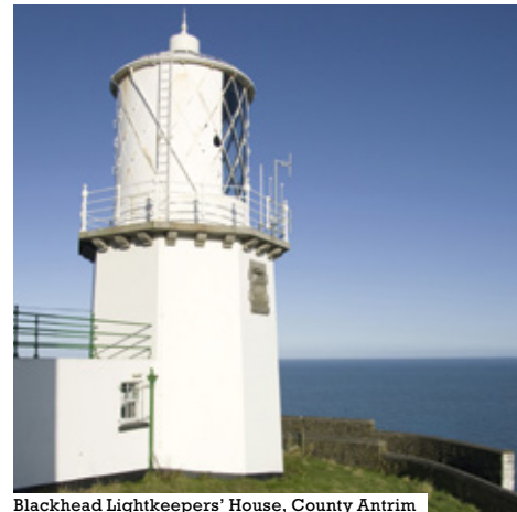
Blackhead Lightkeepers' House, County Antrim
