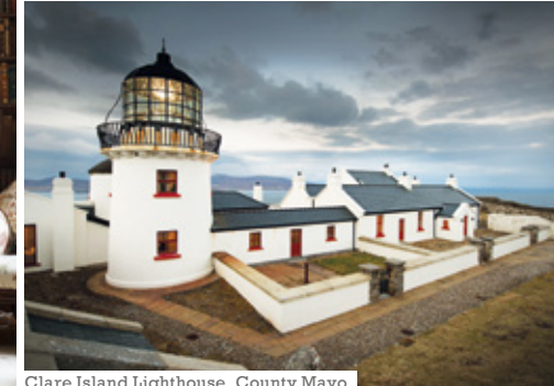
Clare Island Lighthouse, County Mayo
