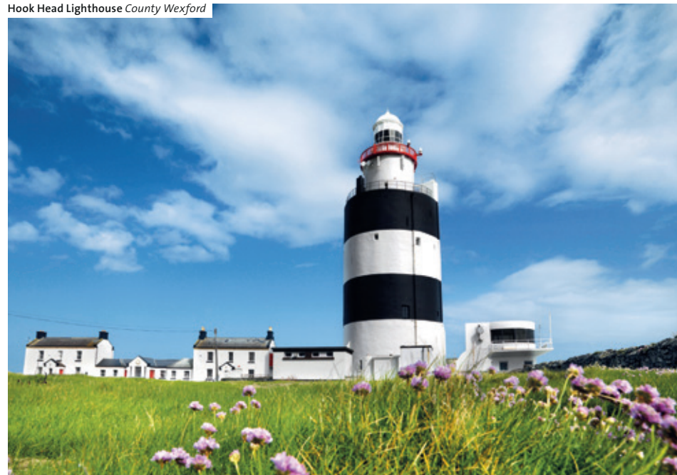
Hook Head Lighthouse County Wexford
