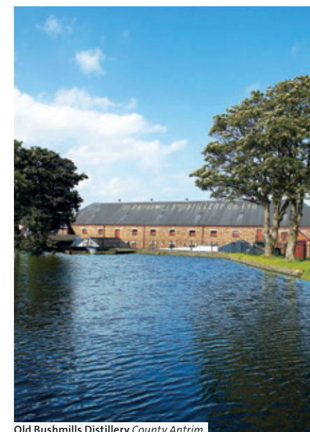
Old Bushmills Distillery County Antrim
