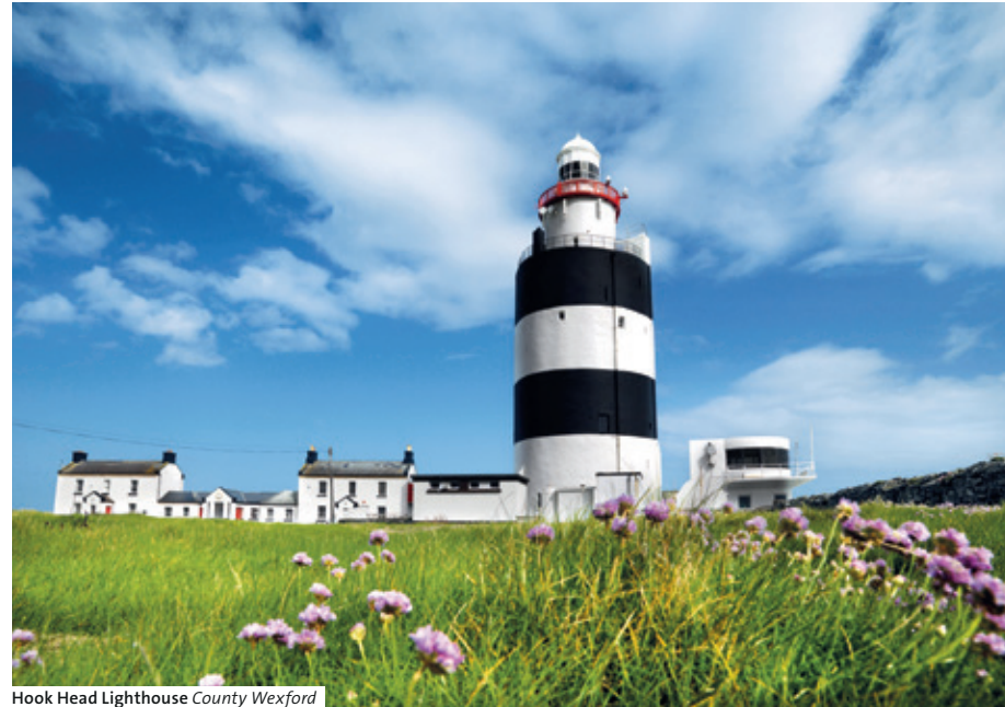
Hook Head Lighthouse County Wexford
