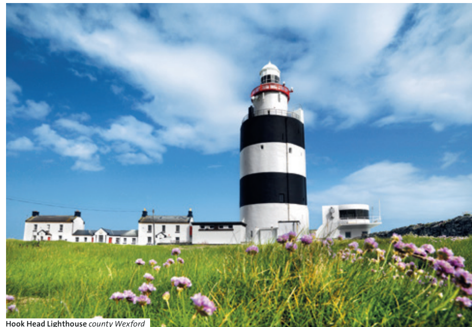
Hook Head Lighthouse county Wexford
